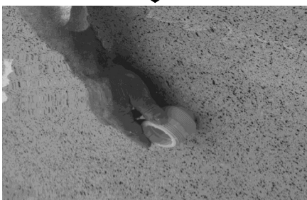
Screw on Insert (3) or (4) firmly
