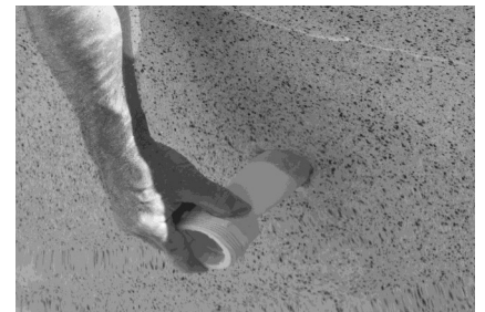
Push in Sanded Insert (1) into hole
