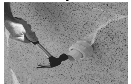
Tap in the Bung (5) into Sanded Insert (1) . This will open the sanded end of the Sanded Insert and secure it to the inside of the pool return.
